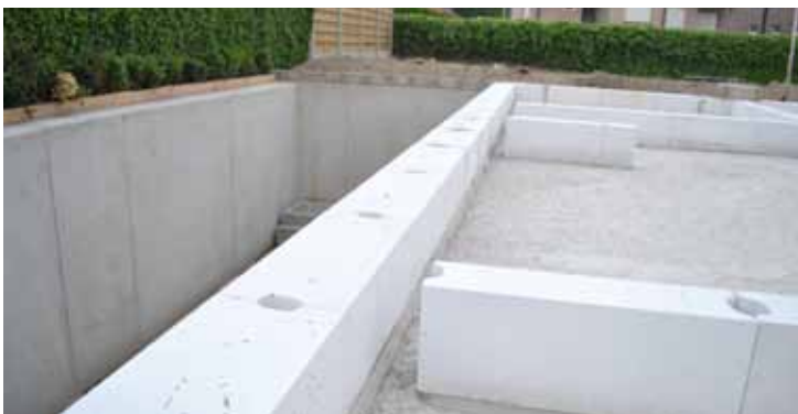
Funderingsaanzet in Ytong
