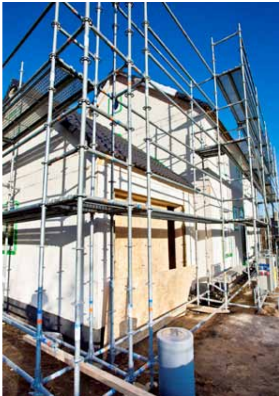
Houtskeltbouw in stelling
